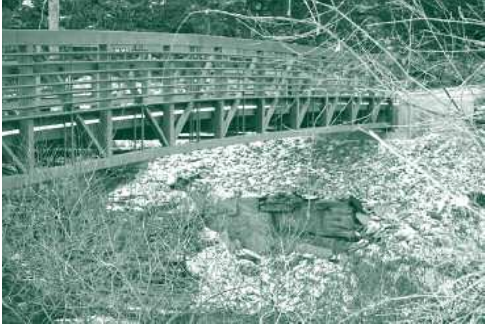
View of the new footbridge (photo: Joe Tierney)
